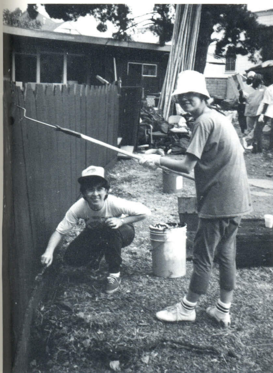
Work progresses at the NAAP work site.
