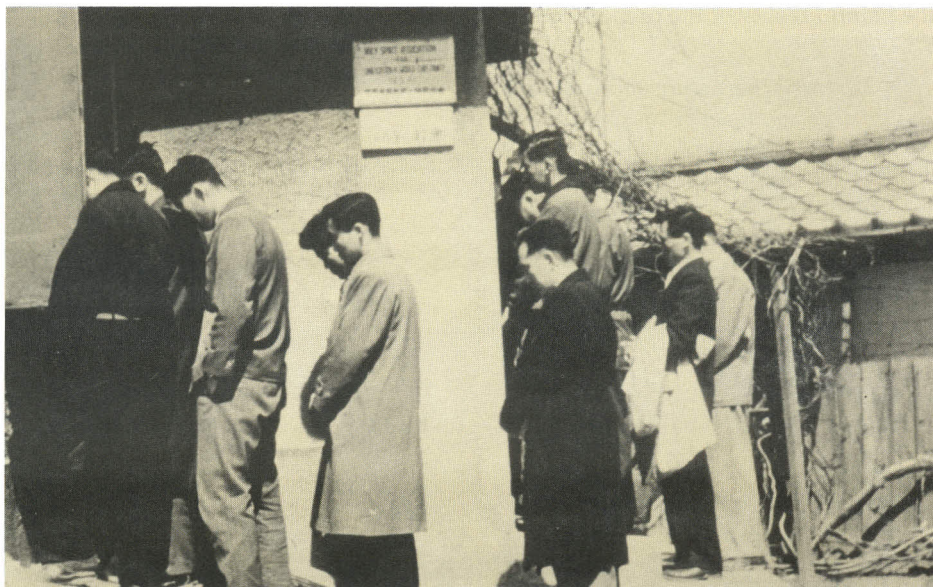
A new foundation, the Unification Church, had to be established.
