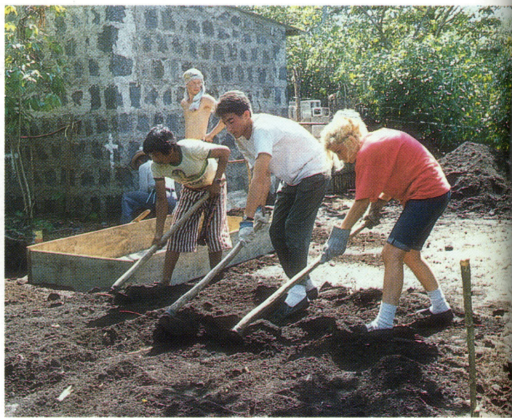
Leveling the foundation for the school.
