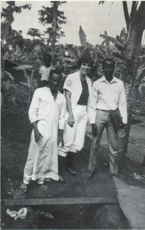
Mrs. Ruth Robinson oversees the construction of new sanitary facilities.
