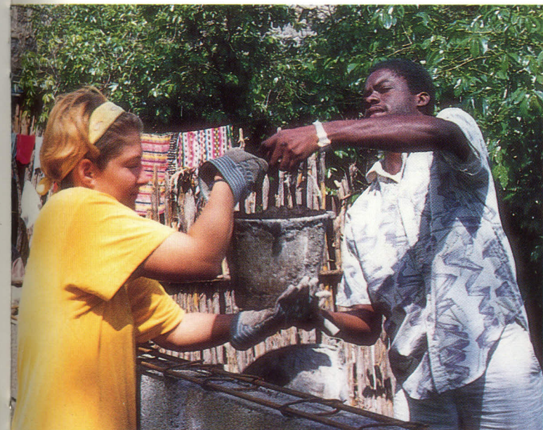
The volunteers participated in every step of the construction work.
