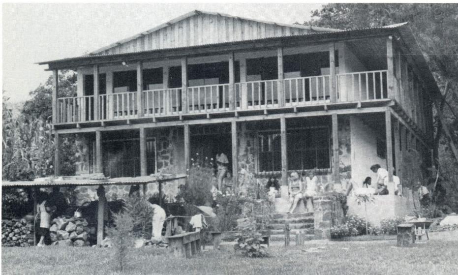
The completed community center built by the WSSC volunteers.
