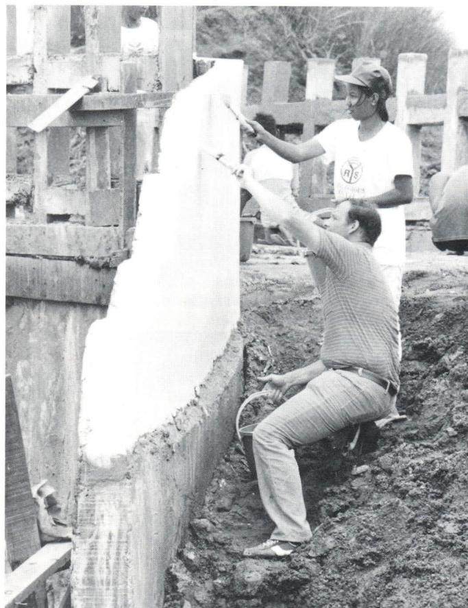
The last finishing touches on the bridge.
