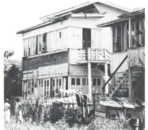
The Joshua House orphanage before restoration.
