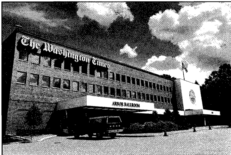
A huge warehouse, formerly the Parsons' paper factory located on the outskirts of Washington, was purchased for the site of the newspaper.
